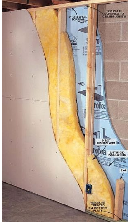
Figure 3-4: Brick Wall with Furring Details
