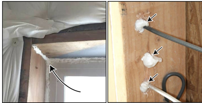
Figure 3-10: Air Sealing
