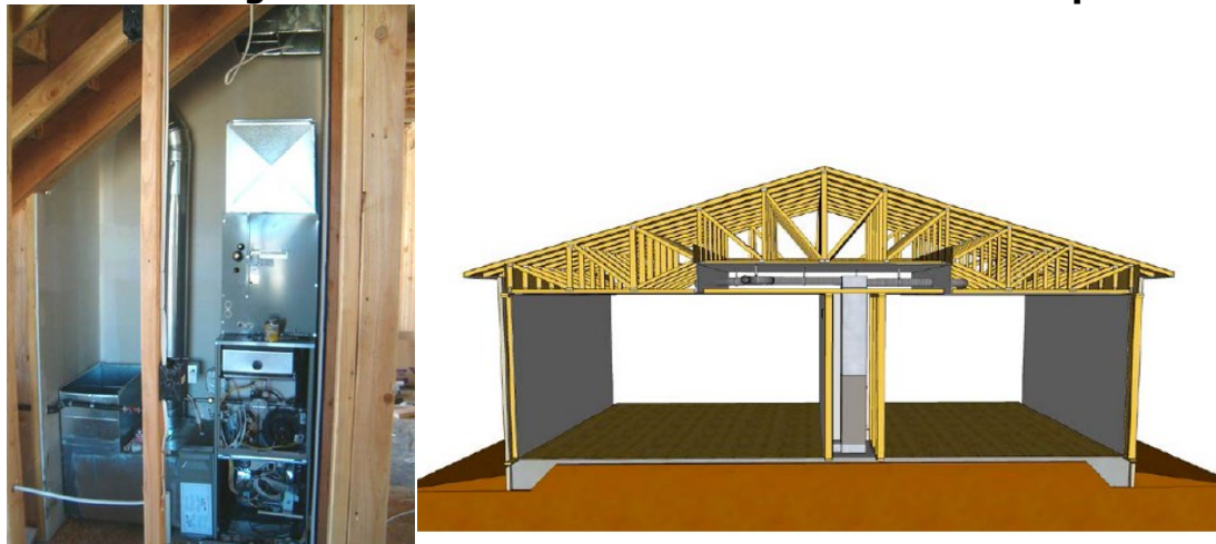
Figure 4-14: Mechanical Closet Placement Example
