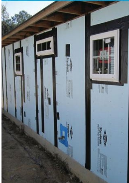
Figure 3-19: Properly Installed Rigid Insulation with Sealant Tape
