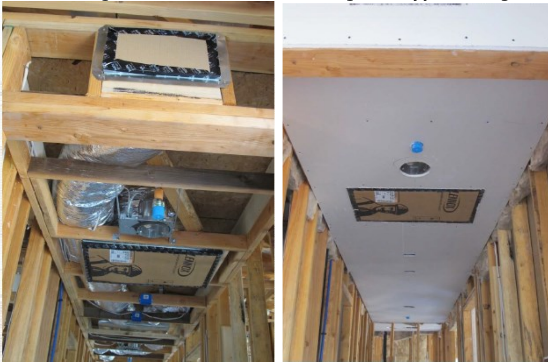
Figure 4-11: Ducts Routed Through a Dropped Ceiling
