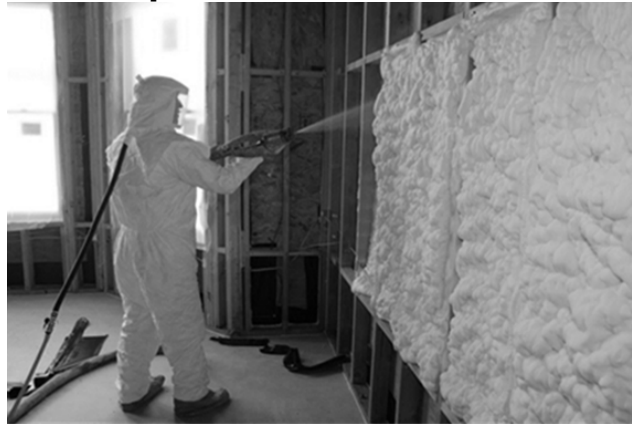
Figure 3-17: Open-Cell SPF Installed in Wall Cavity
