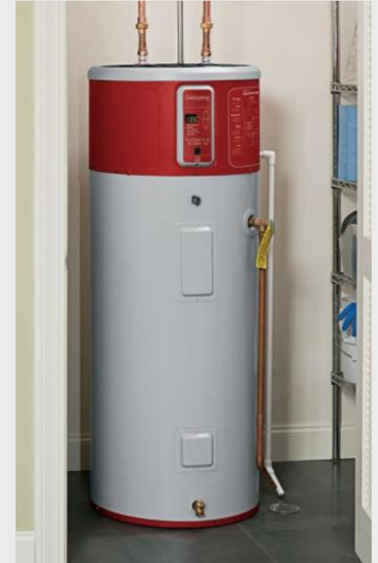
Heat Pump Water Heater
