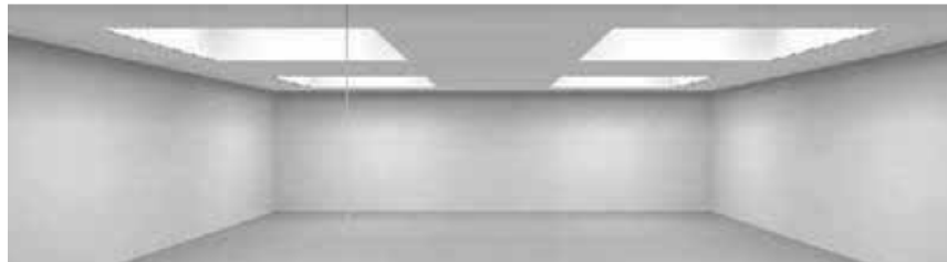
Skylights with splayed light wells
