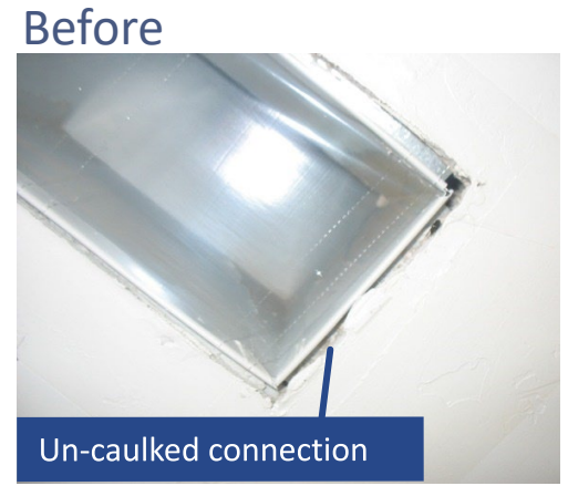
Common Problem Area – Connection to Drywall
