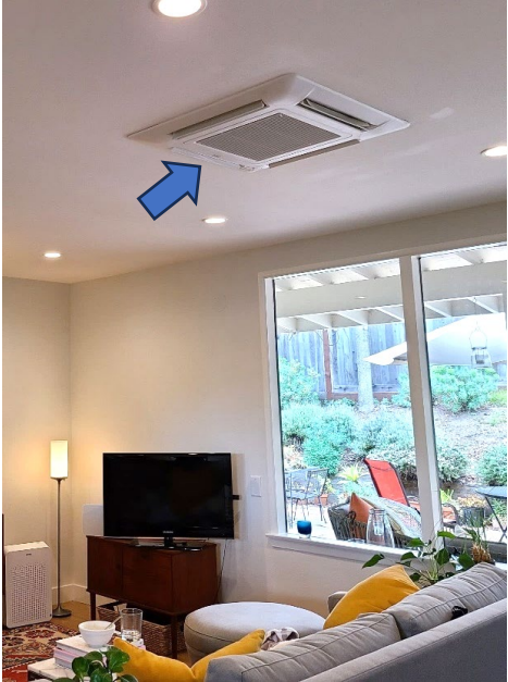
Ductless Recessed-Ceiling
