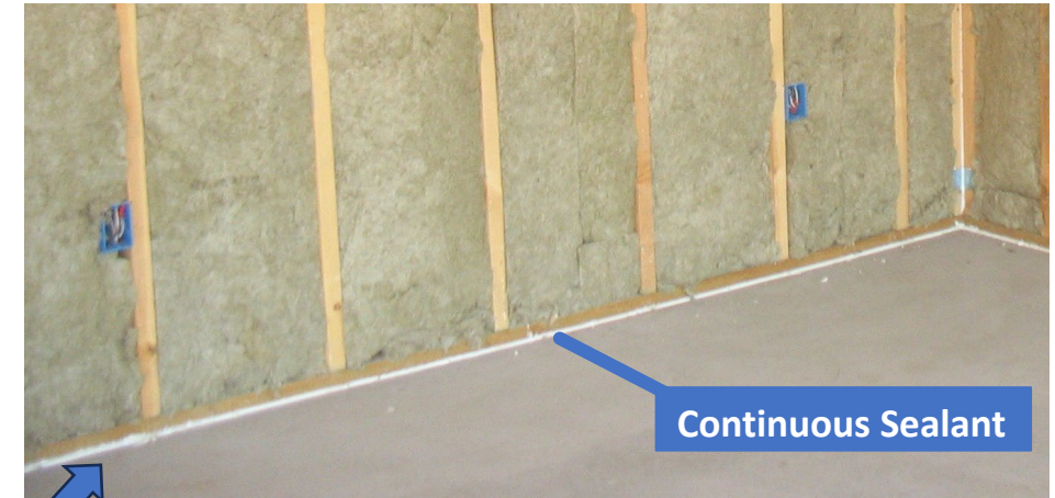
Exterior Bottom (Sill) Plates Sealed to Floor
