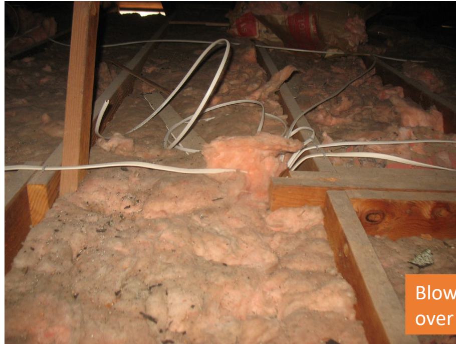
HERS – Verified Existing Condition R-19 in theory, lots of room for improvement
