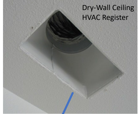
Continuous Bead of Sealant
