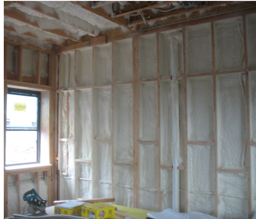
Remaining cavity will be filled with Batt or Blown-in insulation.
