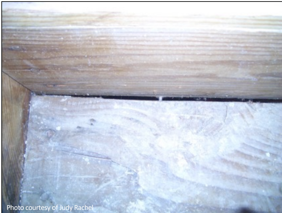
Interior stairs on exterior wall
