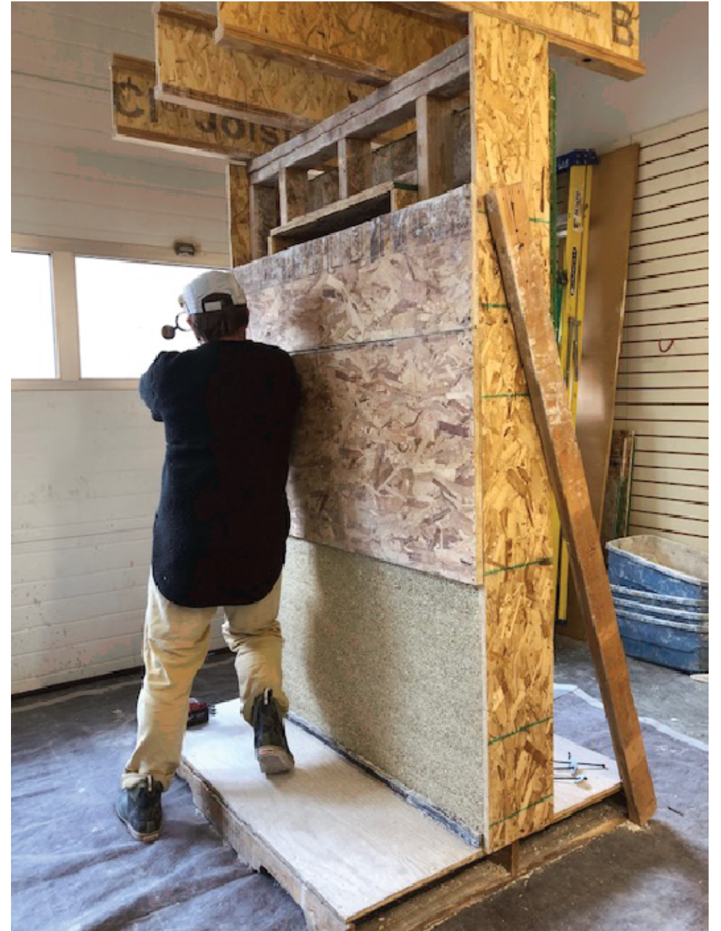
HEMPCRETE FRAME-ON-CENTER WALL CASTING
