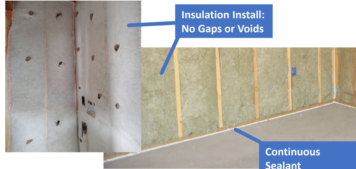
Exterior Bottom (Sill) Plates Sealed to Floor
