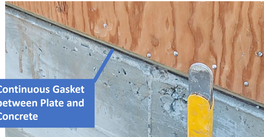
Exterior Bottom (Sill) Plates Sealed to Floor
