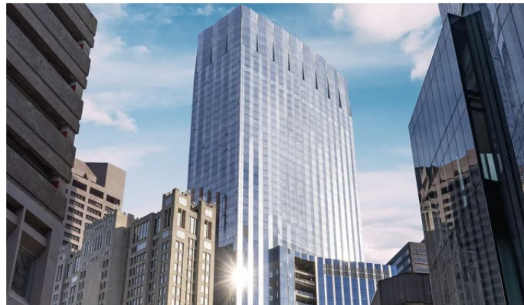
Winthrop Center in downtown Boston is now the largest Passive House office space in the world. (Millennium Partners)
