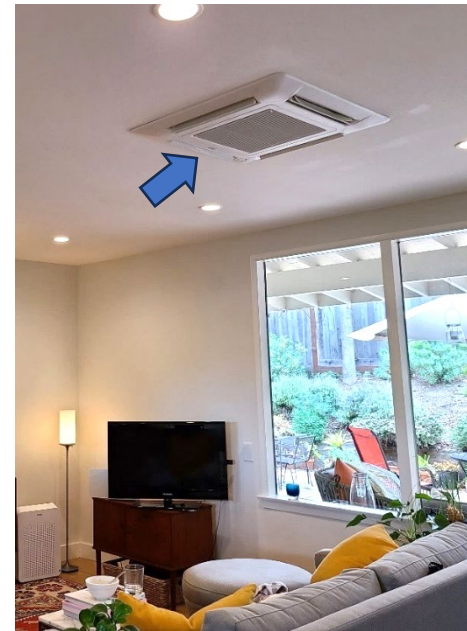
Ductless Recessed-Ceiling
