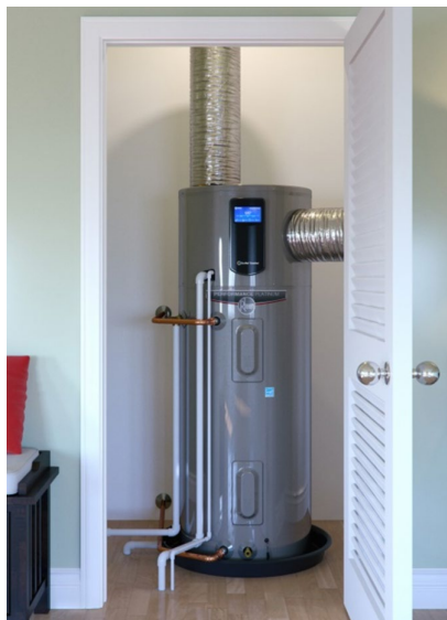
Packaged unit with heat pump on top of tank & ducted to exterior.
