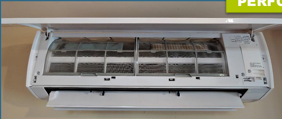
Under the Hood –with clean Filters
