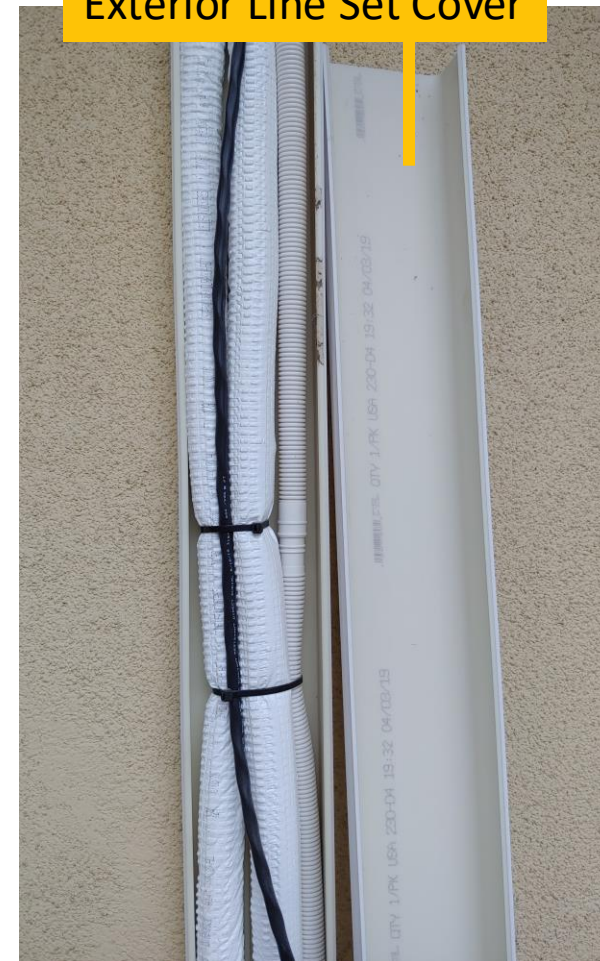
Remodel: Exterior Line Set Cover
