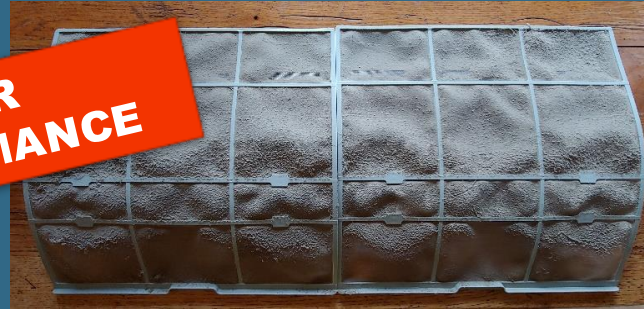
Dirt and Dust Build-up
