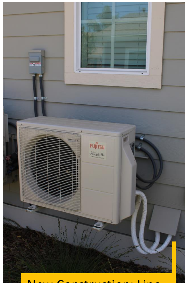
New Construction: Line Set Built-In to Wall
