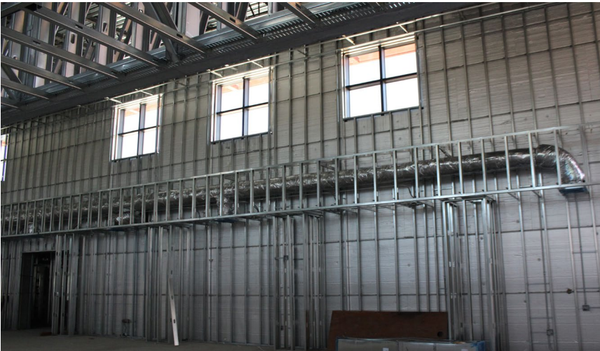
R-10 CI – Held in place with CI masonry fasteners
