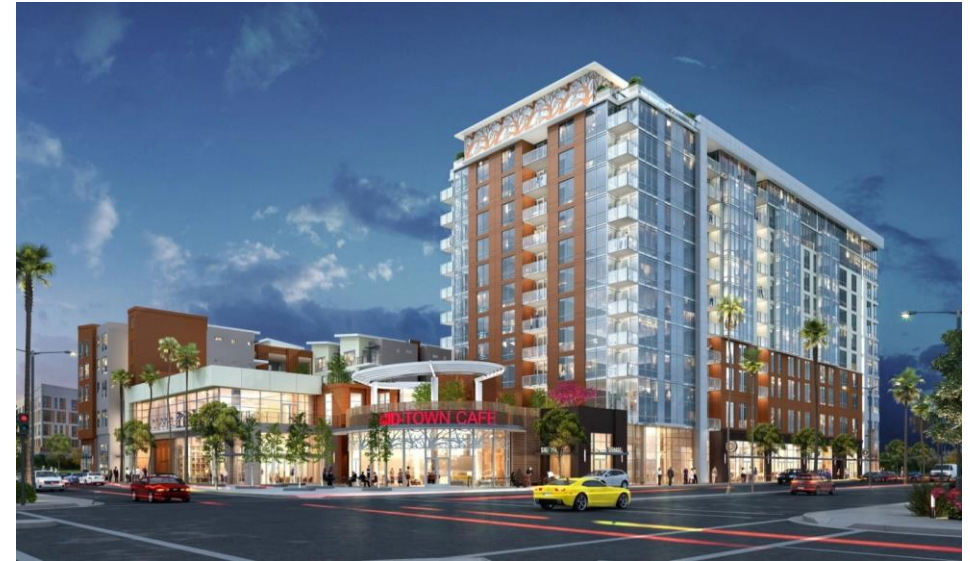
VTA Housing Ohlone Station, San Jose, CA (CZ 4)
